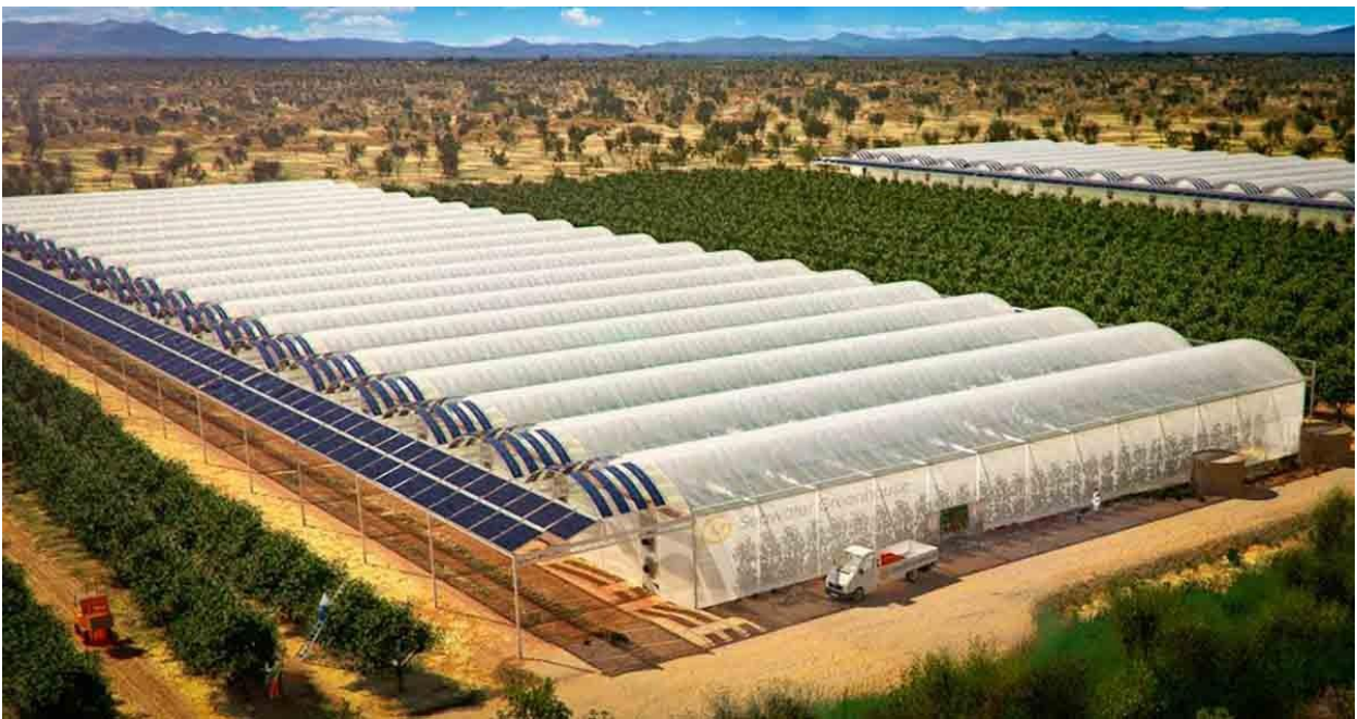
Above – Solar PV provides electricity to polytunnels for food production, storage and pumping water to the crops.
